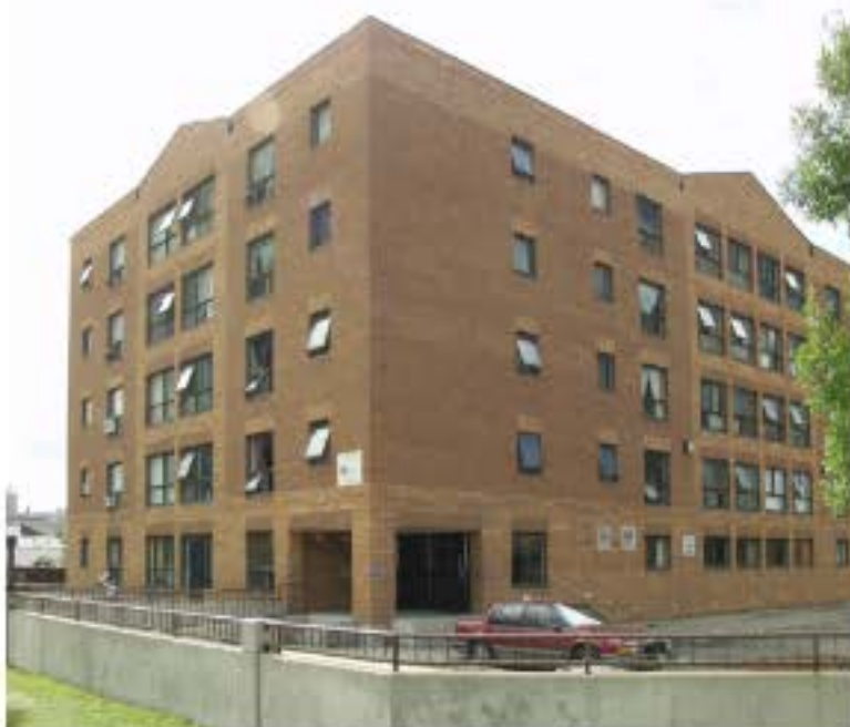
970 Sherbrook Before window replacement
